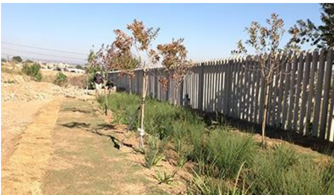
Figure 88. Bioswale in the neighborhood of Diepsloot in Johannesburg, three months after implementation. Credits University of South Africa.
