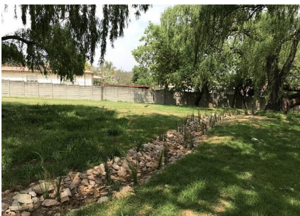
Figure 79. Bioswale in Short Road Park with grasses and stones cover. Credits KH Landscape Architects
