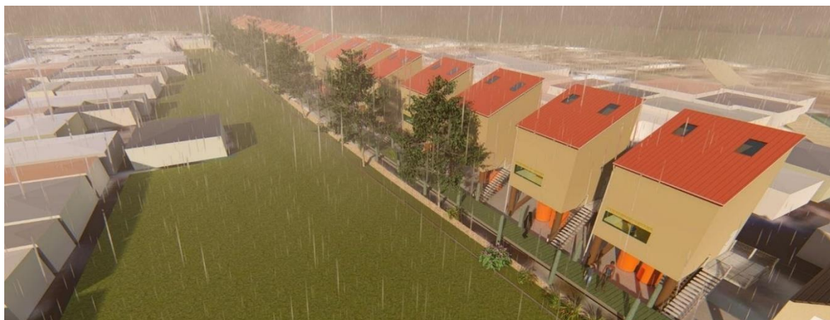
Figure 17. Elevated houses and boardwalks on stilts, elevated refuge site, and bioswale. Elevated houses and boardwalks are encouraged as a solution for areas with a low elevation that are more exposed to floods.
