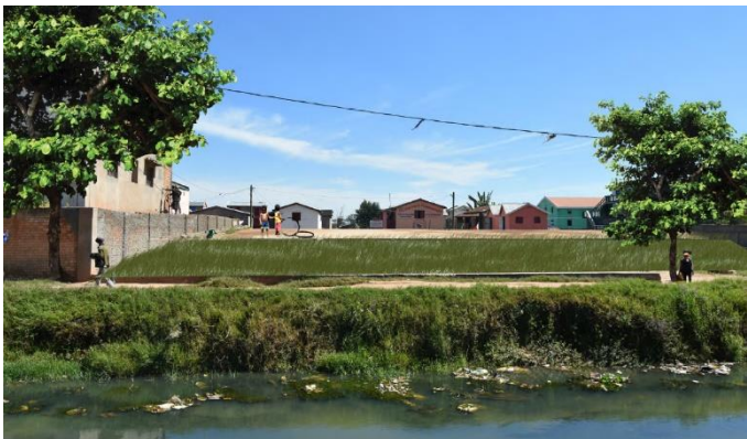
Figure 82. Inspiration image of an elevated refuge site on an embankment over 1m higher than its surroundings.
