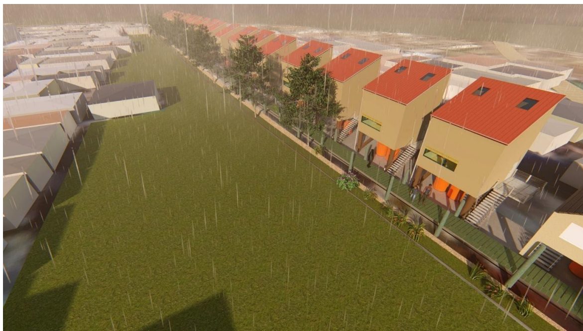
Figure 66. Elevated houses and boardwalks on stilts, elevated refuge site, and bioswale. Elevated houses and boardwalks are encouraged as a solution for areas with a low elevation that are more exposed to floods.
