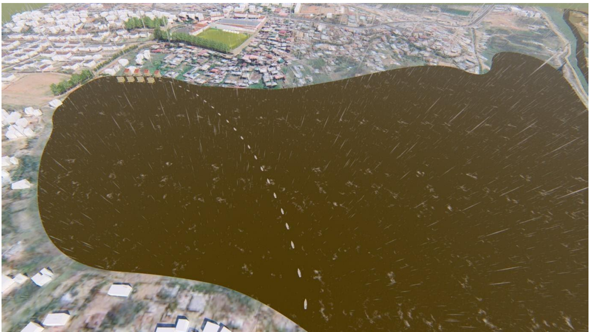
Figure 55. Bird's eye view of site 1 from the south, where the swamp is located.
