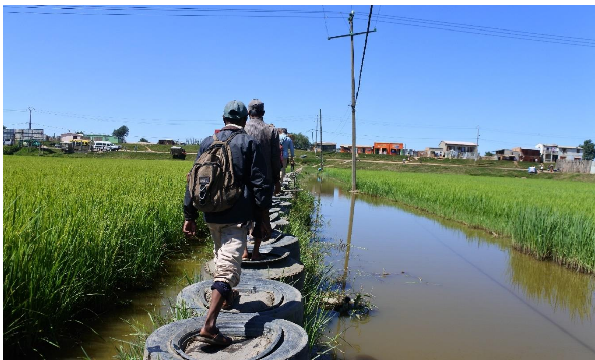
Image 9. Existing elevated pedestrian route
