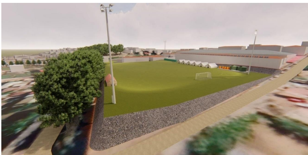
Figure 7. Soccer field as refuge site. The soccer field has been constructed as a terrace on the slope, with its surroundings at a lower elevation, except for the buildings and road on the north.
